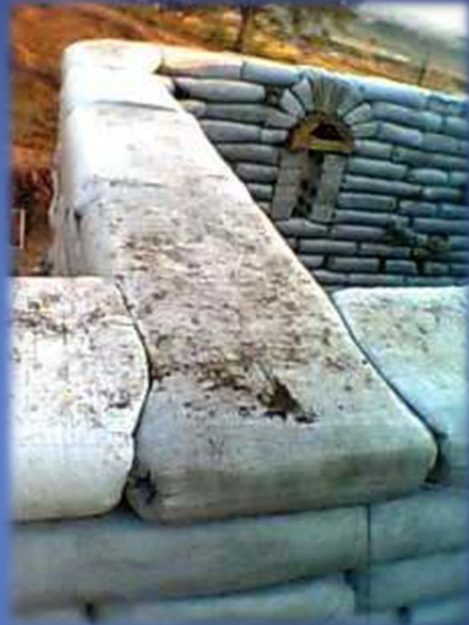
18. Consistent upper row work.
