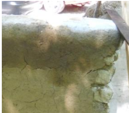
Below: Earthen plaster condition at time of testing
