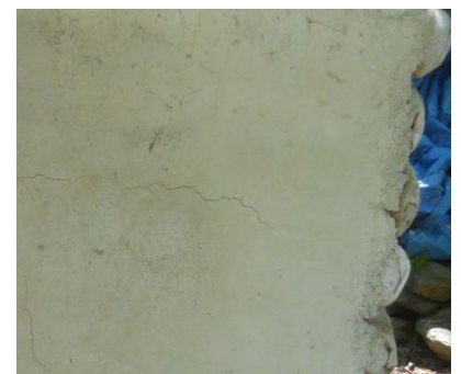
Right above: Lime and earthen plaster side view Right: Lime plaster condition when cured
