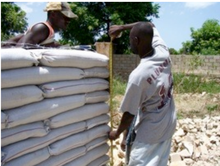
Plumbing and measuring the height of each corner took a little time, but became quicker with practice. It kept our walls coming up straight and even. We tried to tamp to the string plus or minus 2 inches. It doesn't need to be exact.
