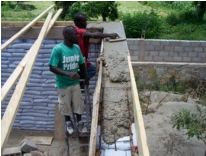
The inside form was made out of scrap wood we had around. It was very twisted and warped, but worked fine.
