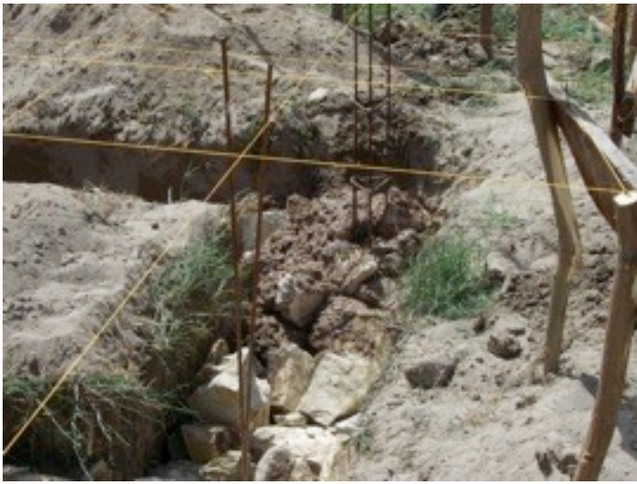
"Rubble" trench served as a foundation. We could have also filled bags with rocks and stacked those to serve as the foundation. I didn't think about it until later. I think I would have put three strands of barbed wire between courses to make sure they "stuck" together.
