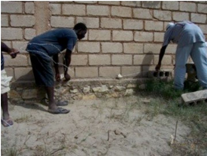
By placing marks along the wall for the different lengths of barbed wire we only had to measure once. We simply cut the pieces as needed and carried them to the wall. It was very fast.
