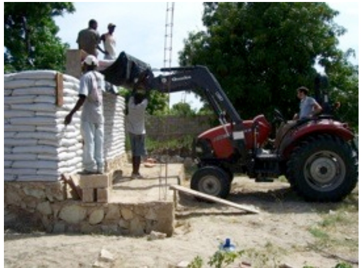
The front end loader on the tractor was nice for lifting a course of bags into place, but not essential.
