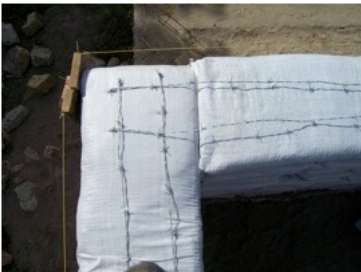
By cutting between the barbs it was easy to poke the first few inches down into the bags and stretch the wire tight.
