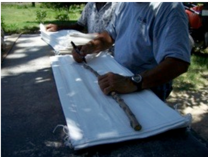
We found marking the bags 6" from the top and filling to that line worked best. We then tamped each course to a line to keep level courses rather than trying to measure the soil.
